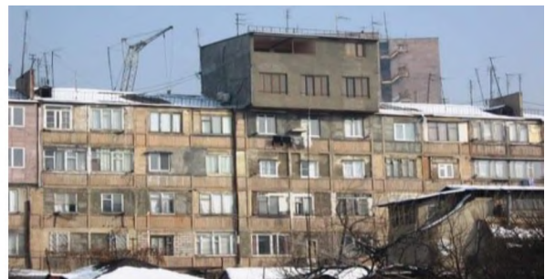
Fig. 2. Added balcony on full height of building
