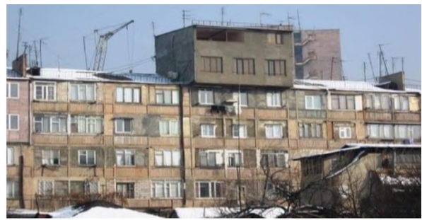
Fig. 2. Added balcony on full height of building
